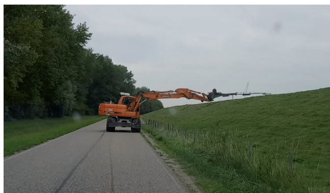
Fig. 2. Sounding of the dam using a crane.
